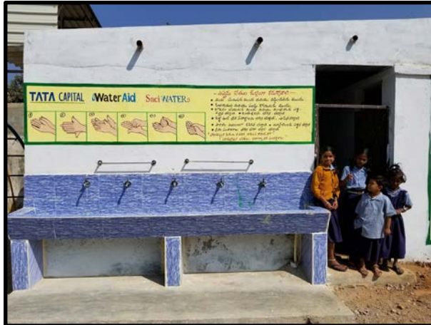
Exhibit 5. SuciWATERS, Water Aid, Tata Capital-funded WASH facility with the six step hand washing process listed above
