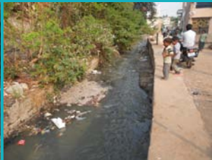
The open drain heading directly to lake
